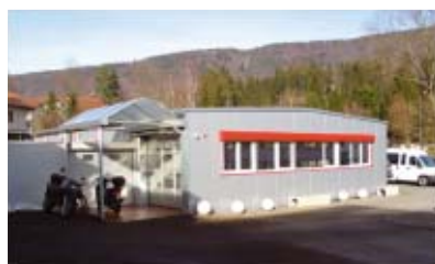
New building for manufacturing steel parts (tool holders, mandrels and accessories).
