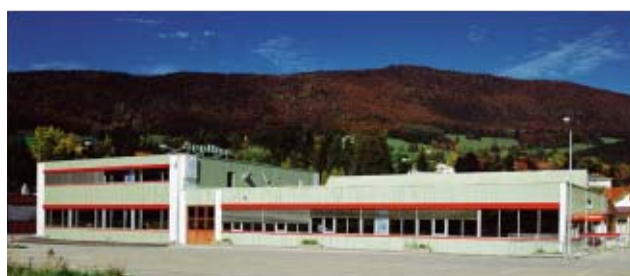
Main building housing the cutting tool production facility, the stores and administrative offices.
