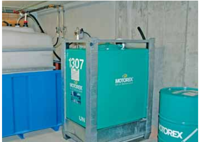
The central machining fluid store in the basement substantially reduces the cost of logistics. Deliveries to and from the store can be made rationally and in full accordance with prevailing safety and environmental standards.
