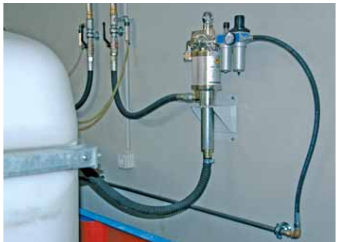
Powerful pneumatic pumps supply the fluid supply column at the central output station in the machine room. Thanks to the universally applicable machining oil MOTOREX ORTHO NF-X, it has been possible to simplify the fluid handling process to a considerable extent.
