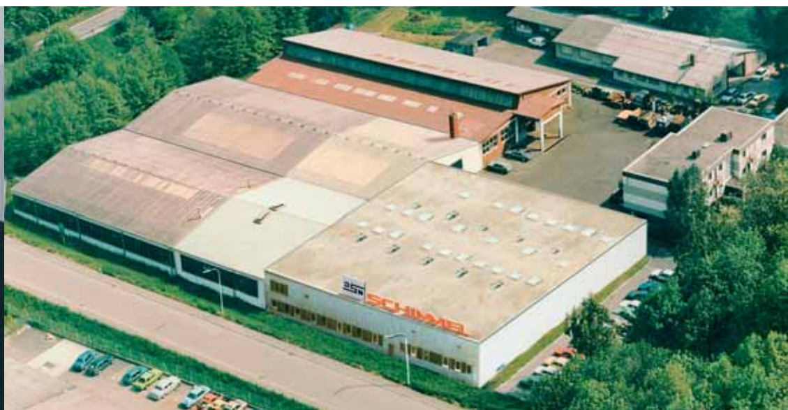
Equipped with high-tech in all areas, the Adelsheim plant now manufactures on a surface area in excess of 15 000 square metres.
